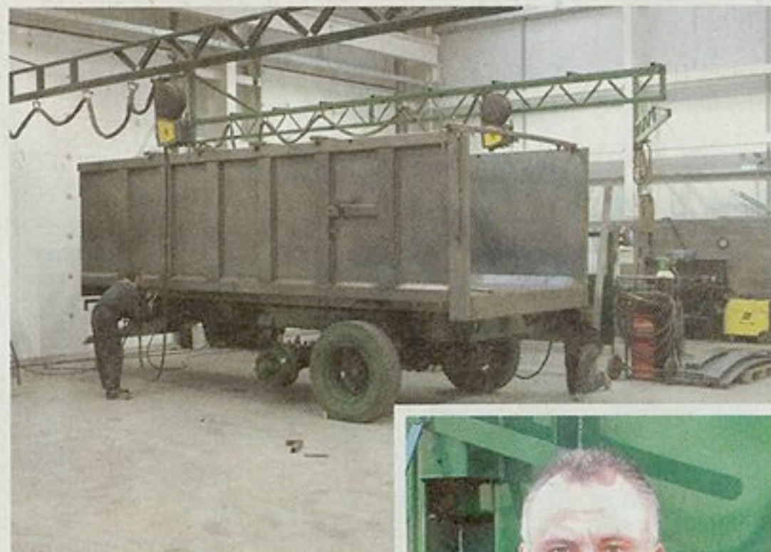
The new factory has four dedicated construction bays where the trailer's floor and sides are added to the chassis and welded up.
